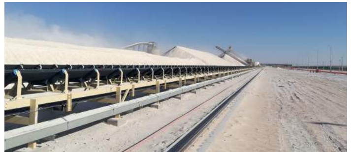
High speed overland conveyor
